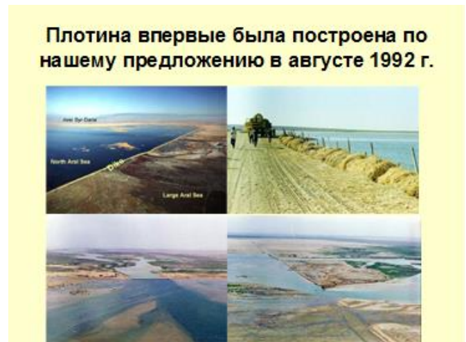
Figure 7: Building of the dam
